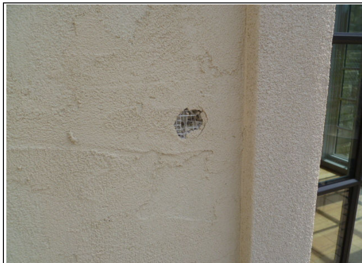
View of damage at EIFS exterior wall material.
