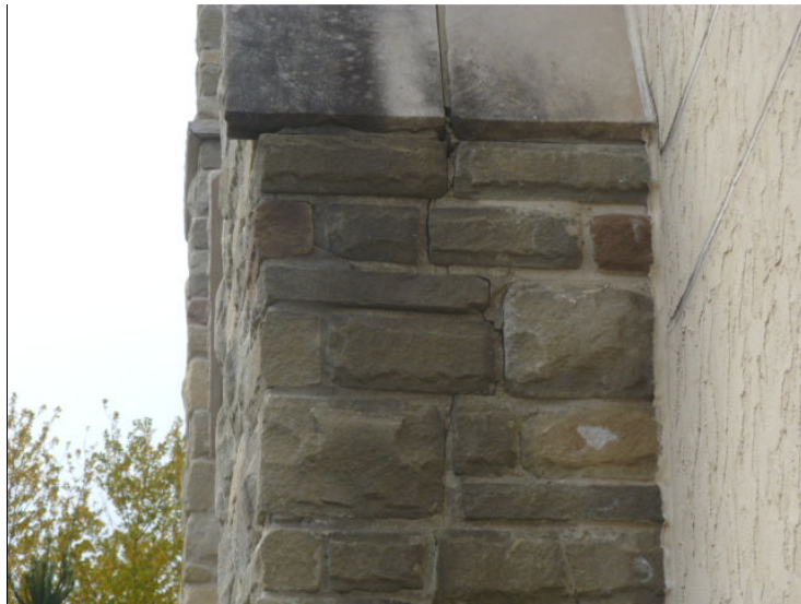
Loose mortar and stone observed on chimneys.
