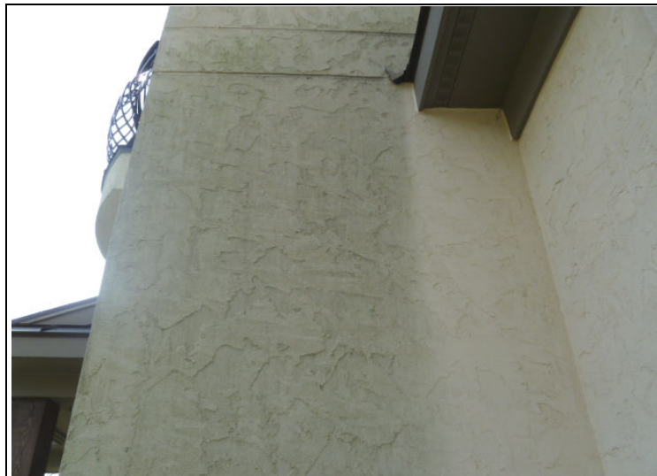
View of water staining on EIFS material.
