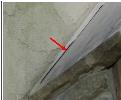
View of decaying caulk at chimney.
