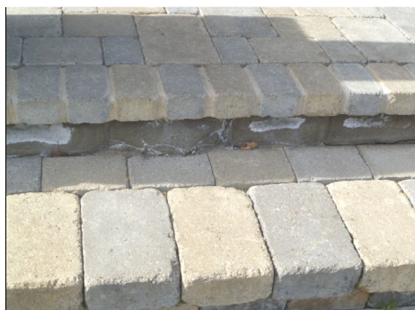
Masonry and mortar decay at front porch.
