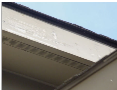
Water damage and exposed wood to fascia board.
