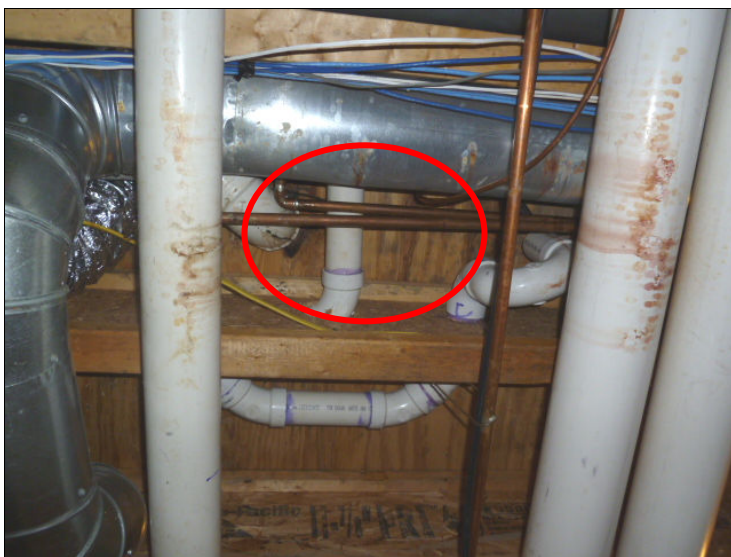
Mold growth on floor framing deck material.
