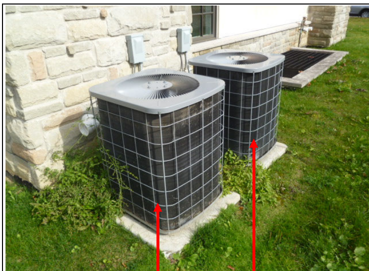
Exterior A/C unit. 2 nd floor unit. 1 st floor & basement unit. First floor unit semi-inoperative.
