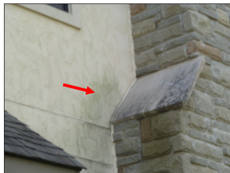
Staining of EIFS at chimneys.
