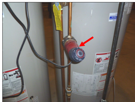
Re-circulating pump inoperative.
