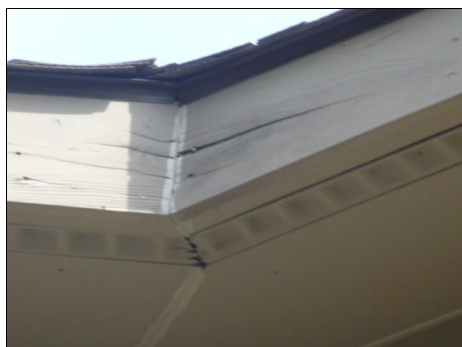
Water damage and exposed wood to fascia board.
