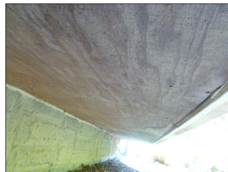
Exposed wood at underside of bay framing.
