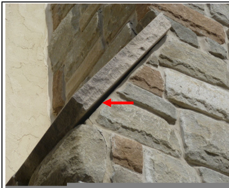
View of loose masonry tile and missing mortar at various areas of chimneys.
