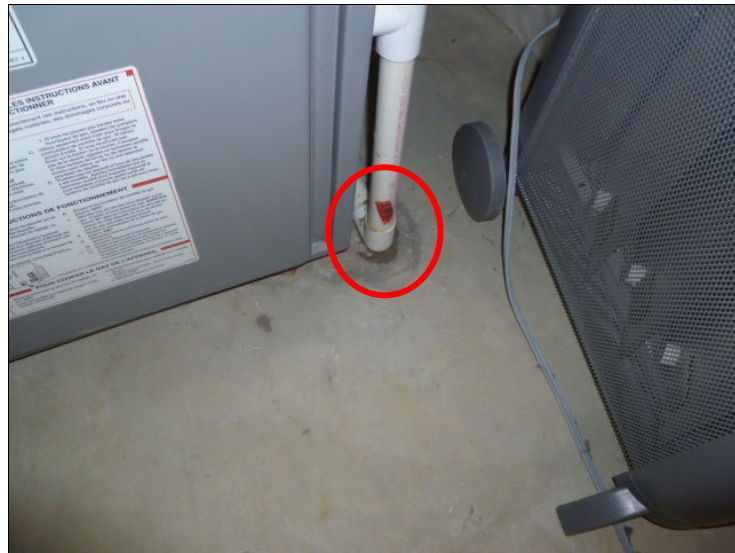
Condensate line leak on 2 nd floor unit.
