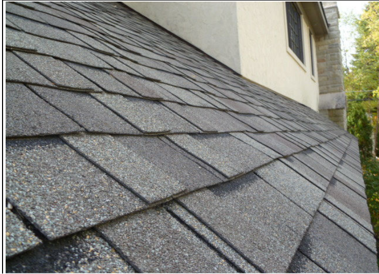
View of asphalt shingle above garage.
