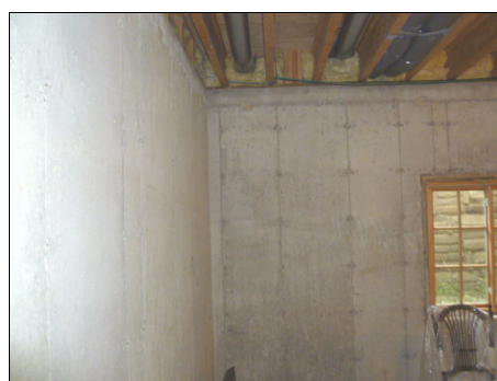
Recommend sealing foundation walls.
