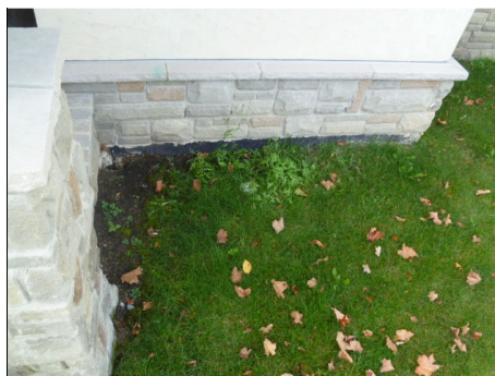
Low grade at front wall.
