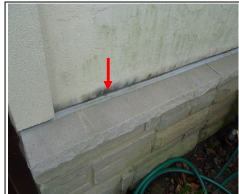
EIFS water damage at sill.
