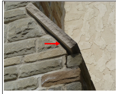
View of loose masonry tile and missing mortar at various areas of chimneys.
